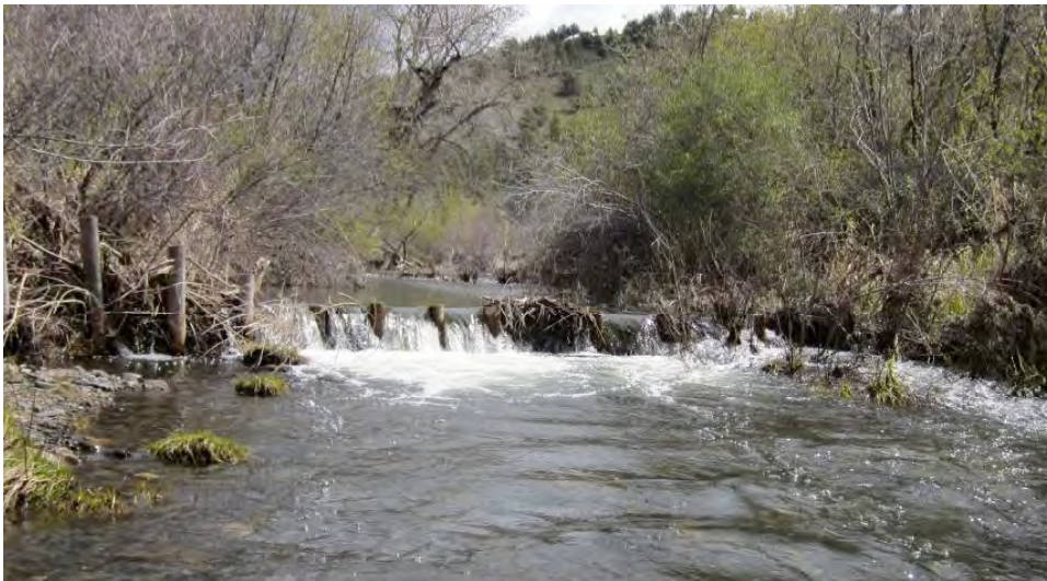
Figure 5. Photograph of a beaver dam analog structure.
